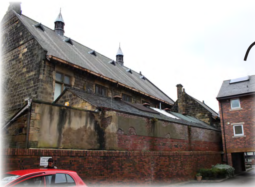
The wall and roof of the 1893 extension are in poor condition, seen here from The Shires car park. (Accessed with kind permission of Yorkshire Housing).
