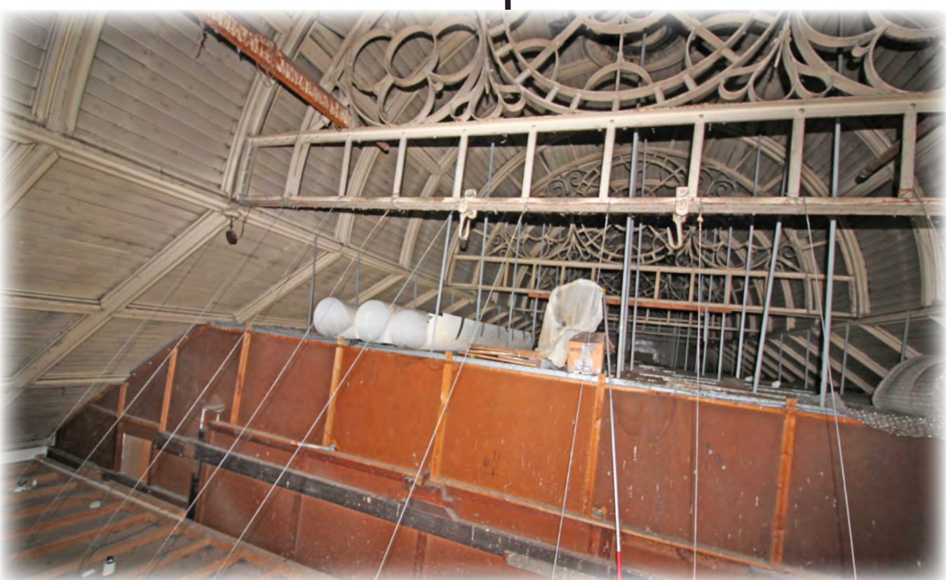
The original decorative iron trusses of the main hall, hidden away above a suspended ceiling. They were manufactured by Dawson & Nunneley of Hunslet, Leeds.
