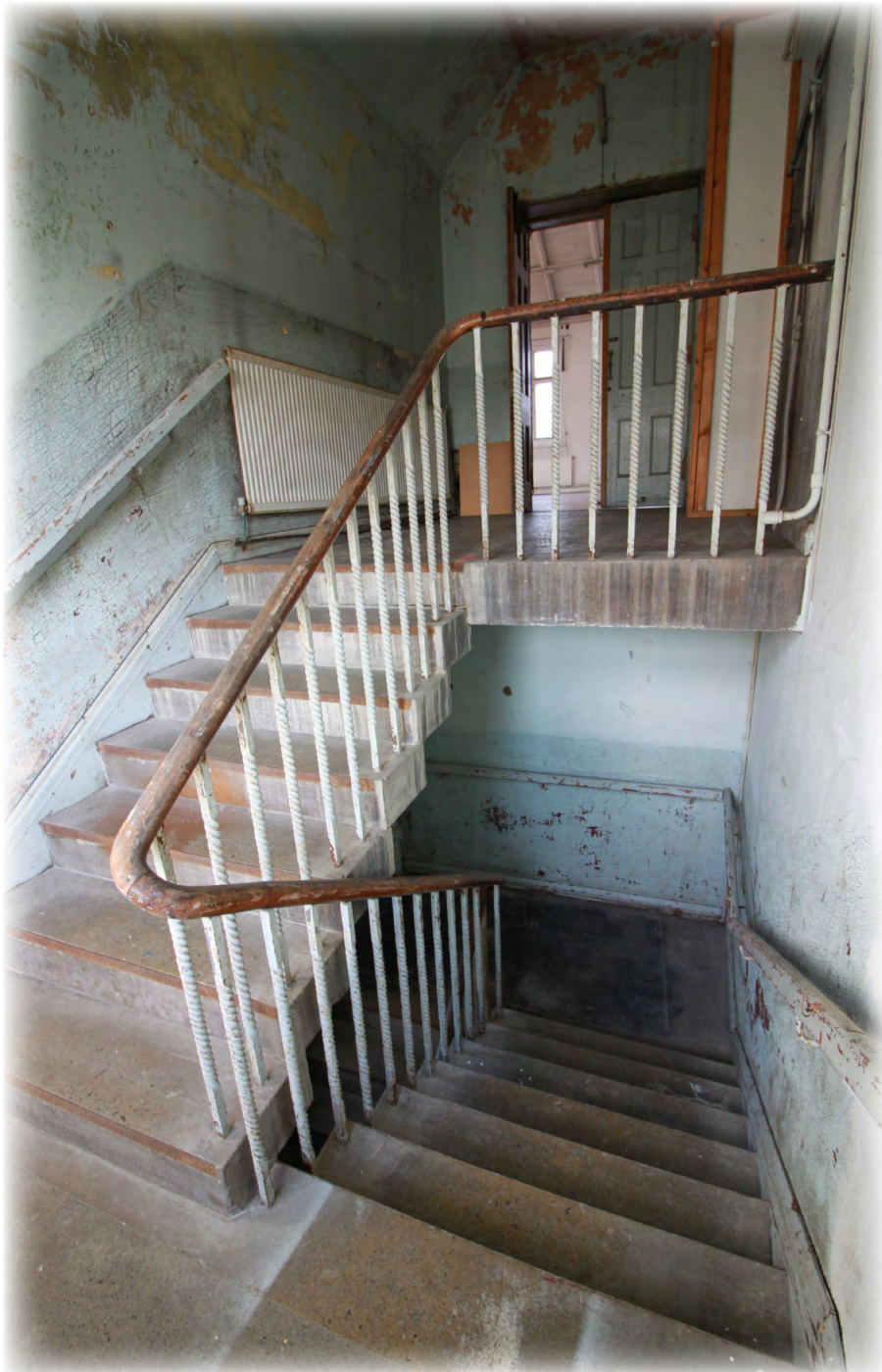
The beautifully simple back staircase with concrete treads, twisted wrought iron balusters and mahogany handrail. The rail to the landing is too low to be safe guarding against fall and the gaps between the balusters are above 100mm, meaning a child's head could get stuck between.
